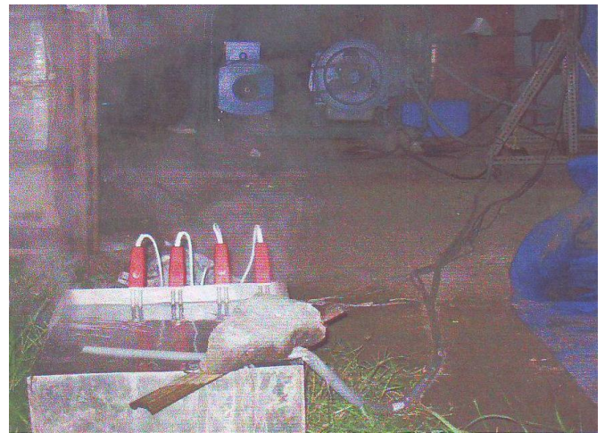
Figure 3. Instalation of Diesel Engine With Electrical Loads
